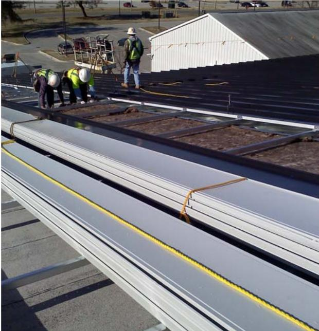
**Figure 2 Solar Air Heating Roof Installation**
