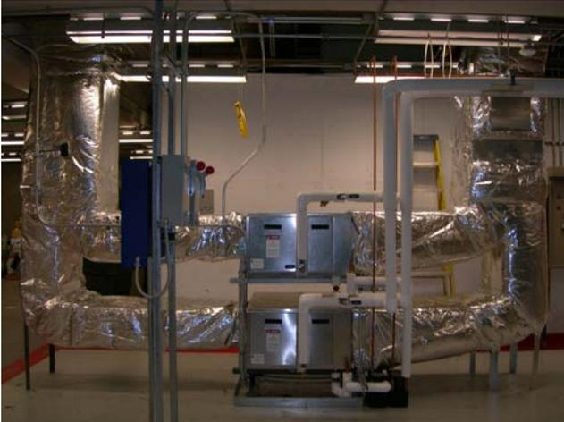
**Figure 1 HHS Heat Pump Heat Recovery System**
